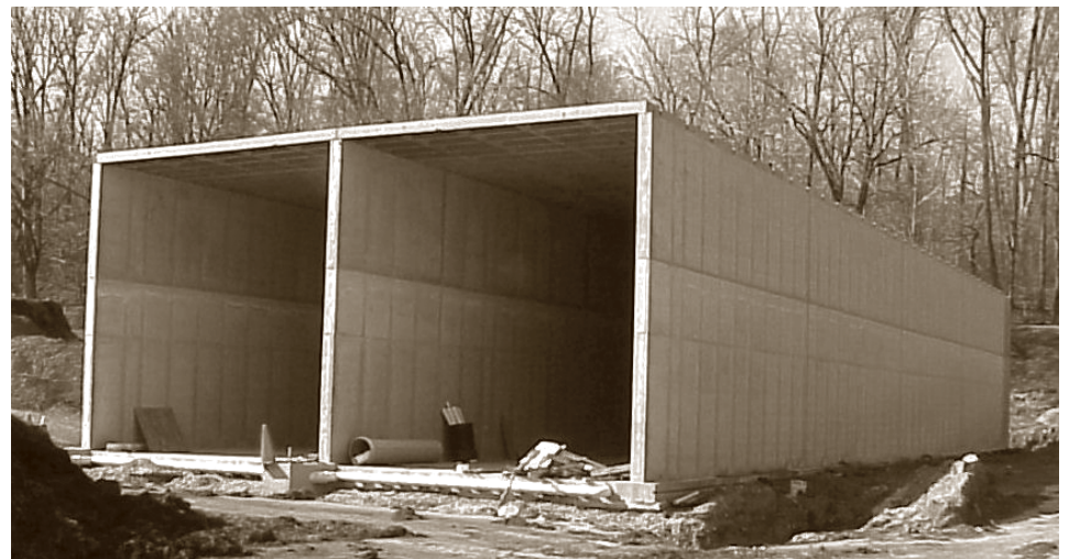
Figure 5. Forced-aeration composting bunkers under construction.
