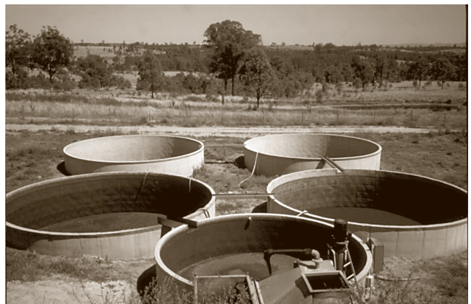
Figure 6. Holding tanks for substrate leachate.
