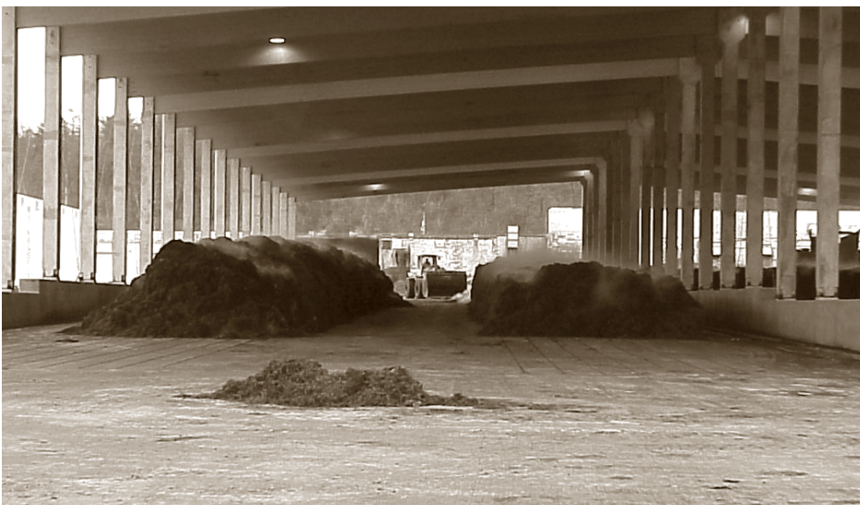
Figure 2. Substrate preparation with a covered roof.
