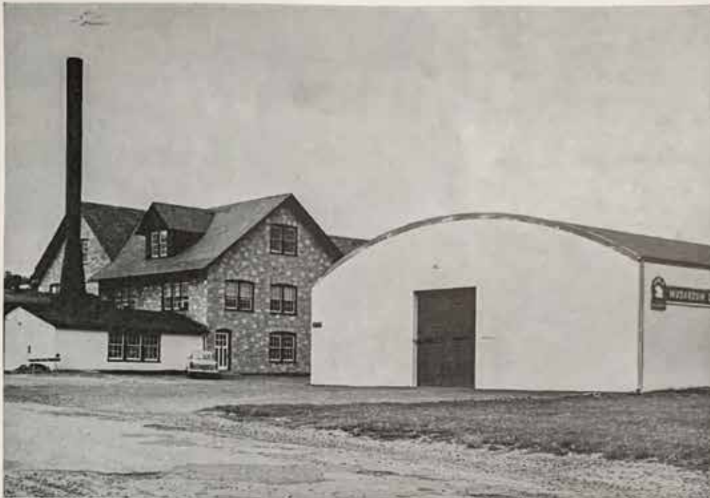
Mushroom Cooperative Canning Company is one of the oldest canneries in the industry. This view shows the main plant and, in the foreground, part of the company's warehouse in Kennett Square.
