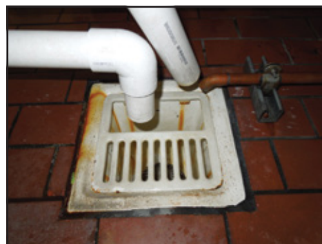
Condensation and drip pan drainage lines and floor drains are common risk-based swab sites for environmental test monitoring programs.
