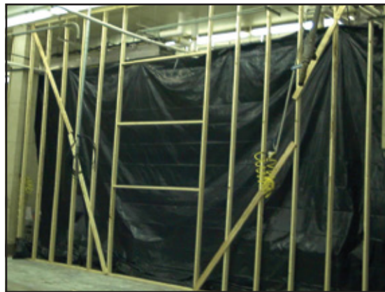
Temporary barriers can protect the production environment from aerosols and traffic that may carry Listeria exposed during construction.
