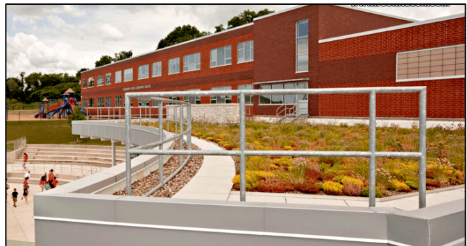
Selinsgrove Elementary School – Selinsgrove, PA
